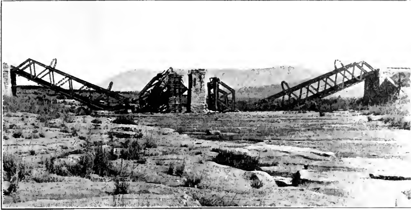
THE RAILWAY BRIDGE AT WASCHBANK (NATAL), BLOWN UP WITH DYNAMITE BY THE BOERS.
